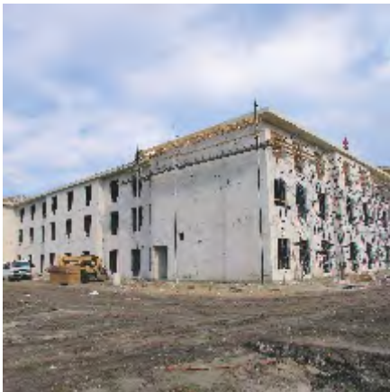
Fig. 22: Three-story hotel construction.
